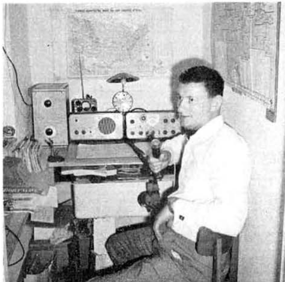
ZB2AO in Gibraltar runs a Courier CTR-1 transceiver into a TA-3 and an end fed wire. The operator, Dick, holds the call G3PLL
